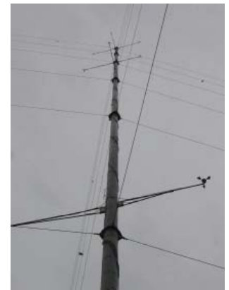
A meteorological tower was used to explore the potential for commercial wind energy production on Bellingham's waterfront
