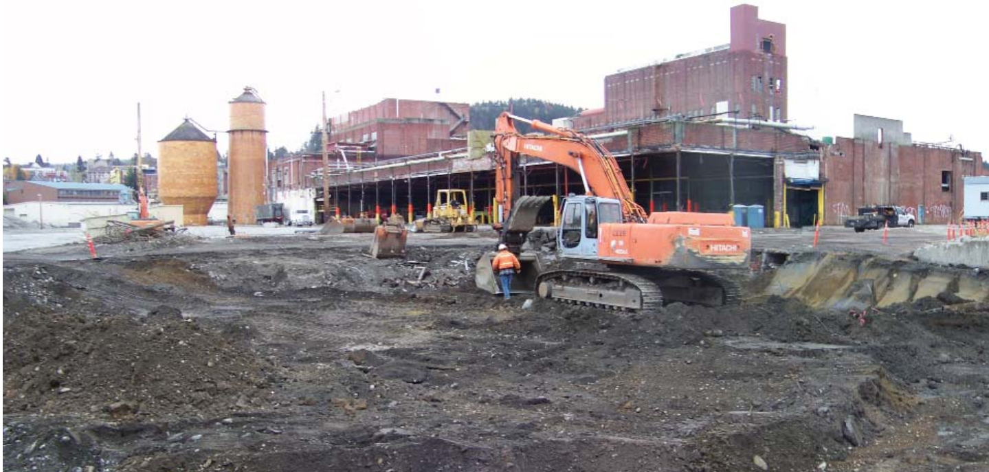
The cleanup of a Bunker C tank on Bellingham's central waterfront in December 2011
