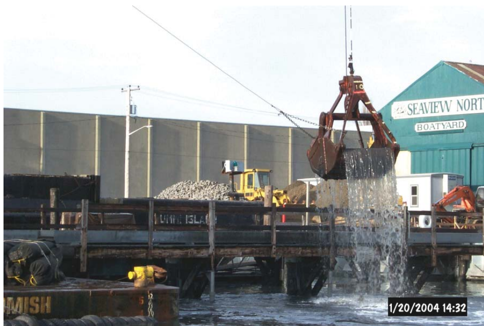
Contaminated sediments are removed from the Weldcraft boatyard
