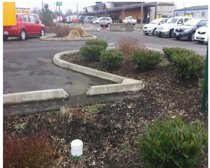
A low impact development rain garden is used to manage stormwater at the Bellingham Airport
