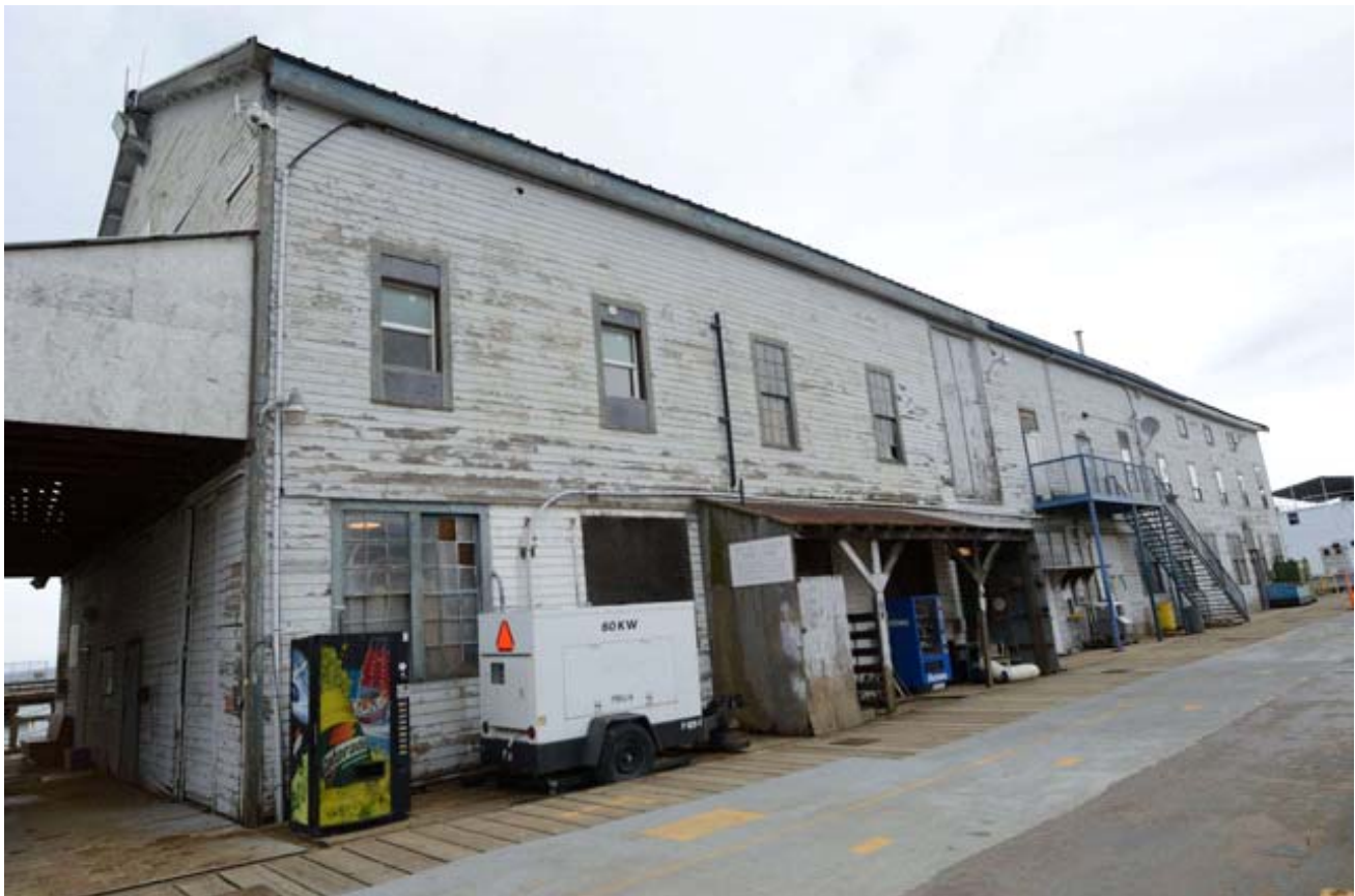
10. East Elevation, View Northwest
