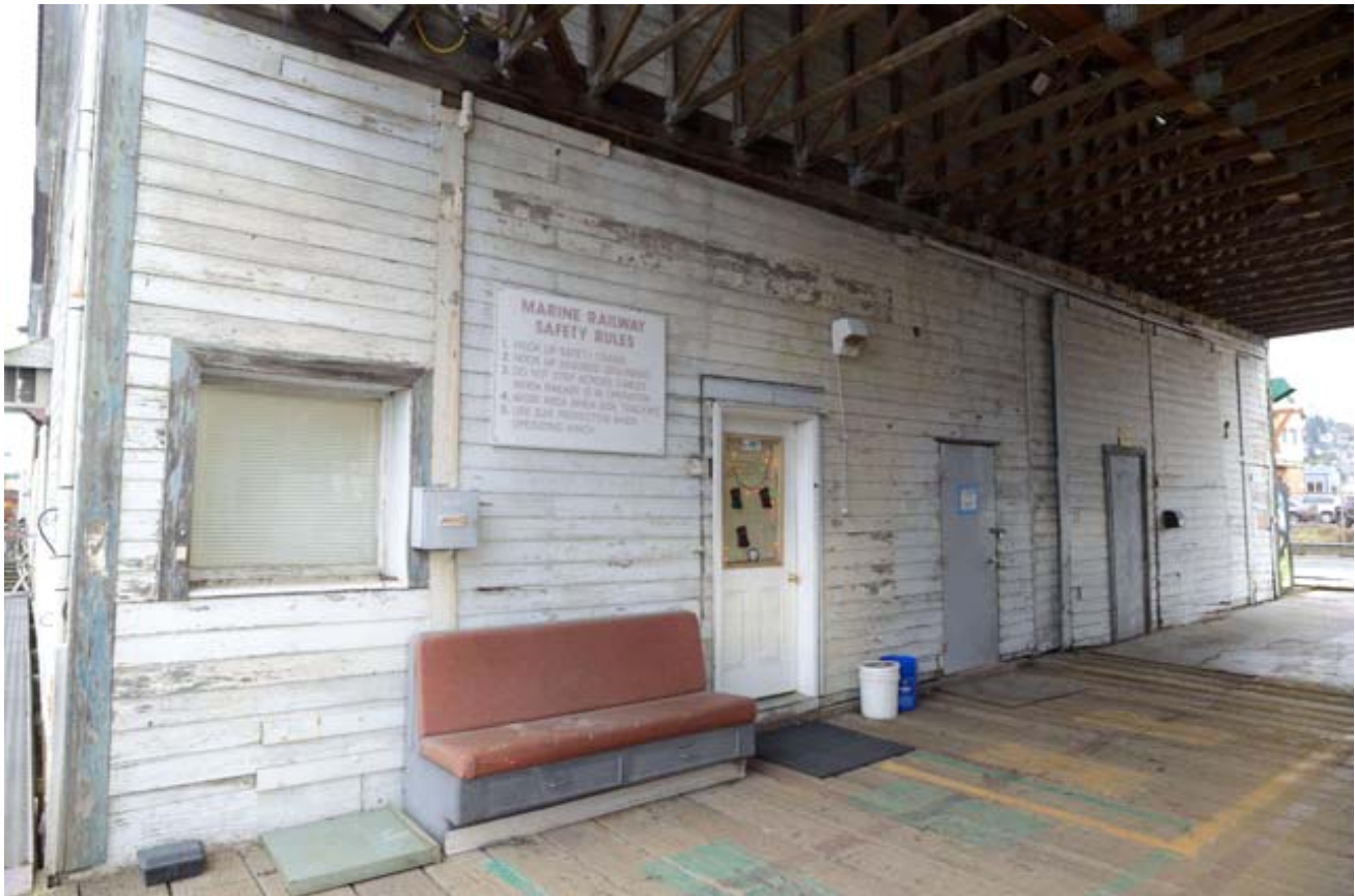
17. Detail of South Elevation, View Northeast
