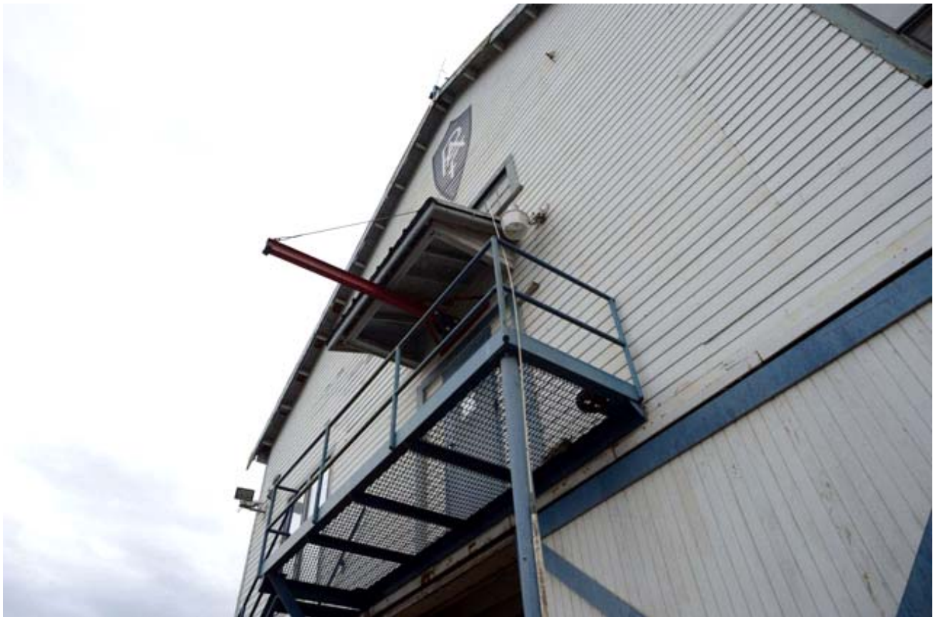
4. Detail of North Elevation, View Southeast
