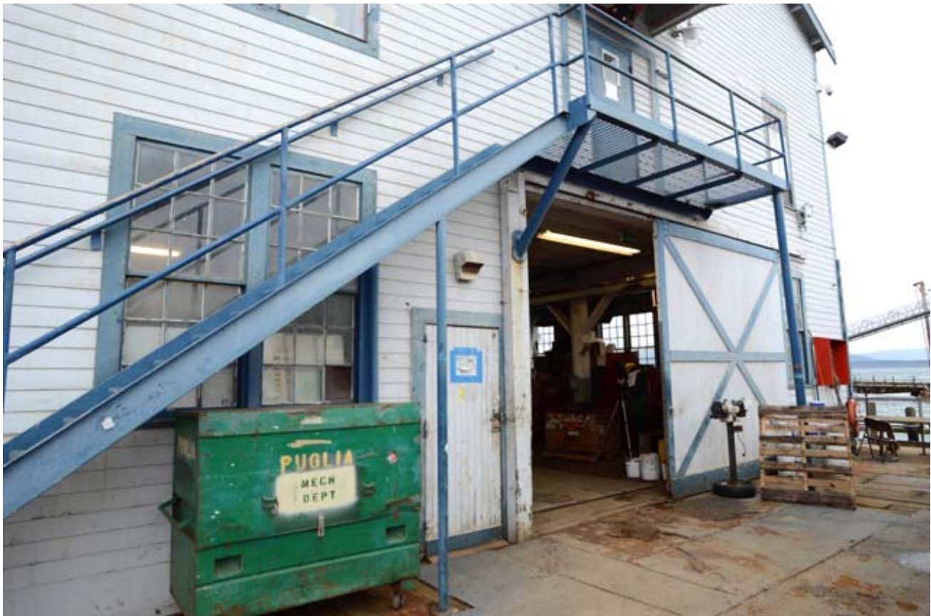
2. Detail of North Elevation, View Southwest
