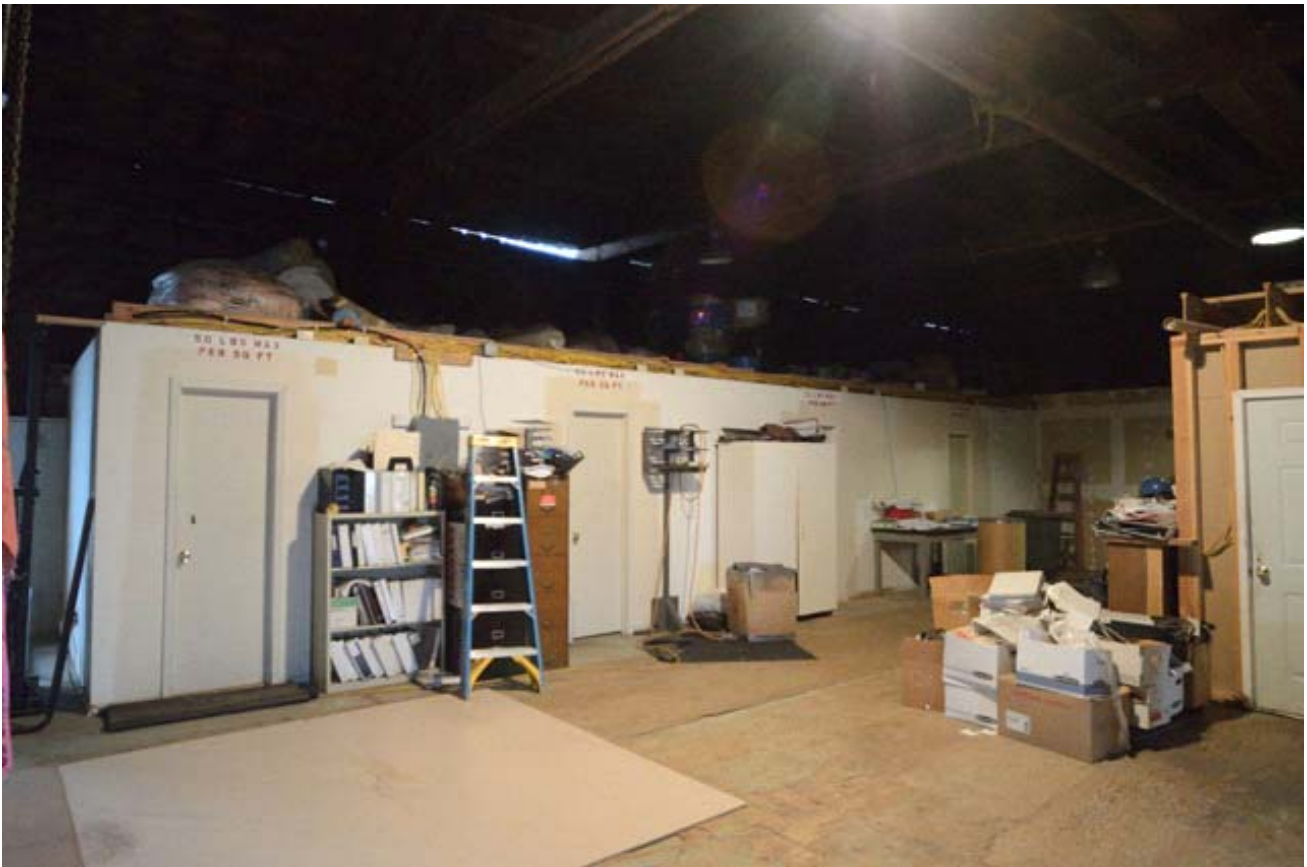
59. Second Floor, Storage Area, View Northwest
