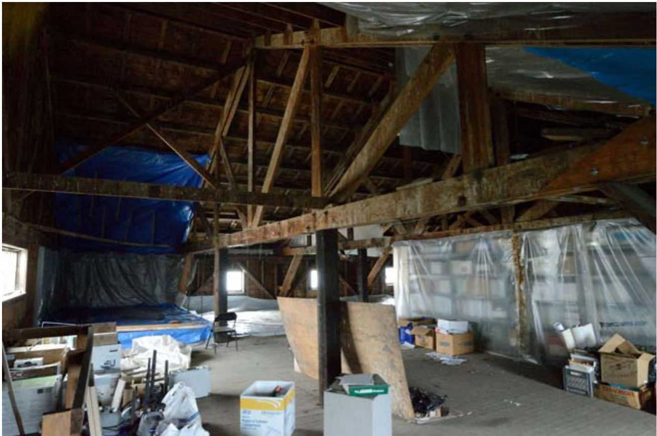
61. Third Floor, View Southeast
