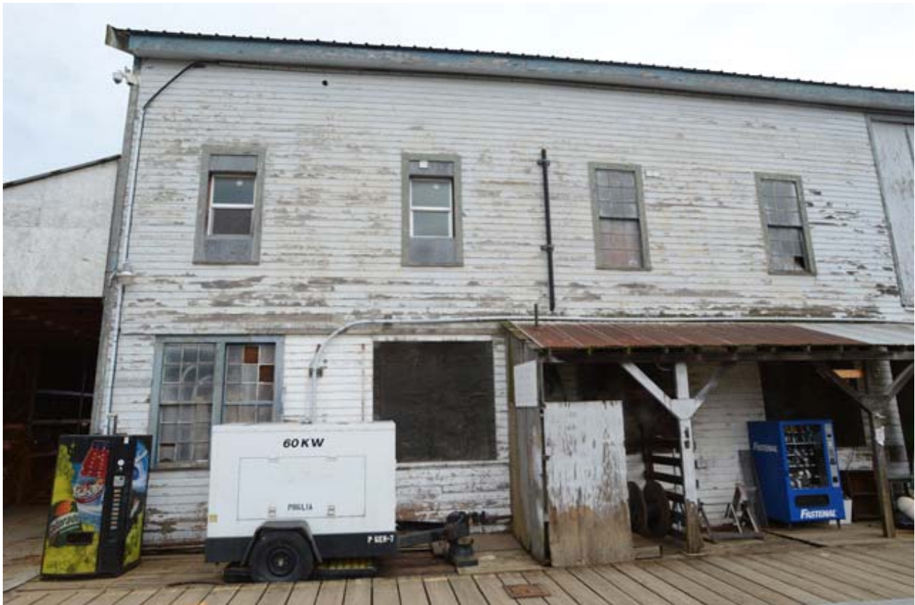
9. Detail of East Elevation, View West
