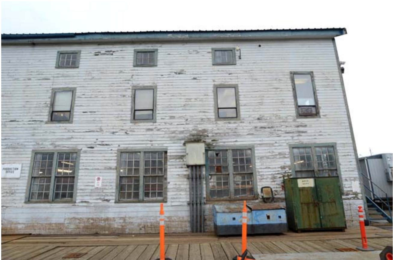
5. Detail of East Elevation, View West
