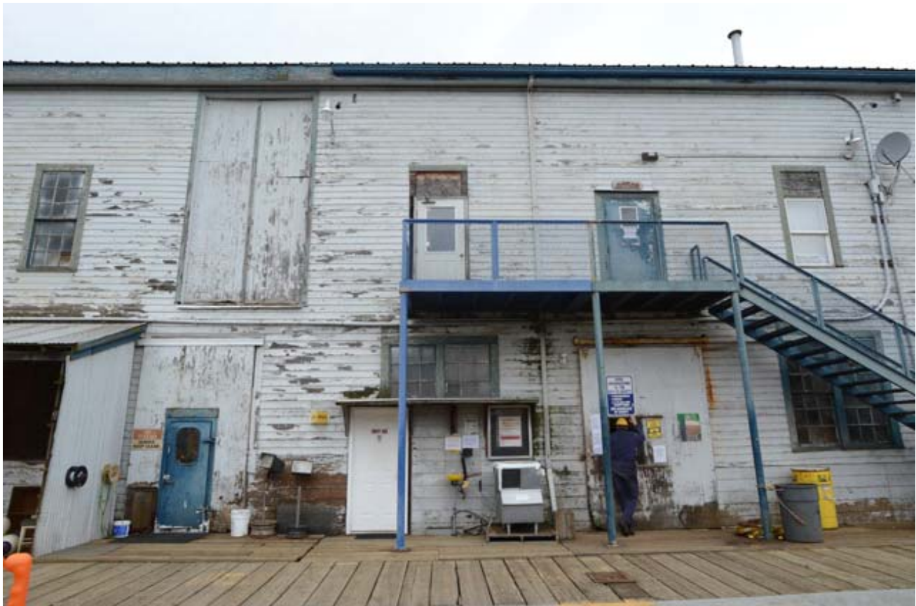
7. Detail of East Elevation, View West
