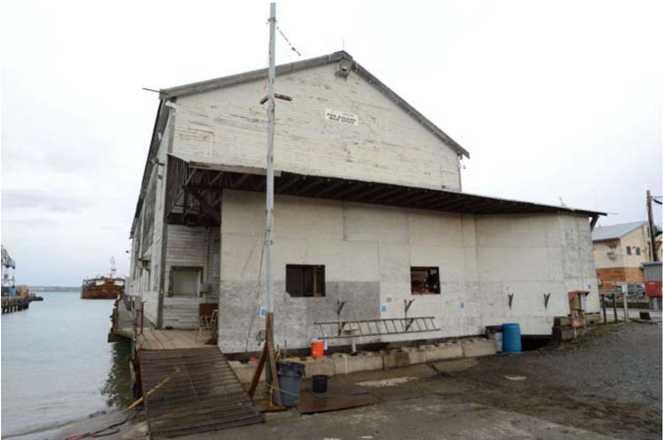
14. South Elevation, View Northeast
