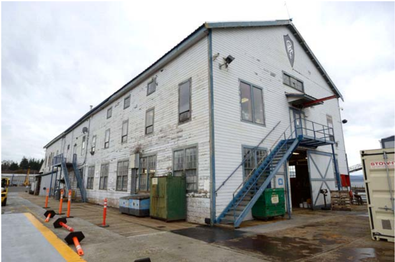
1. North and East Elevations, View Southwest
