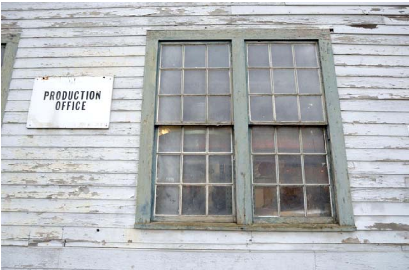
18. Detail of Window, East Elevation
