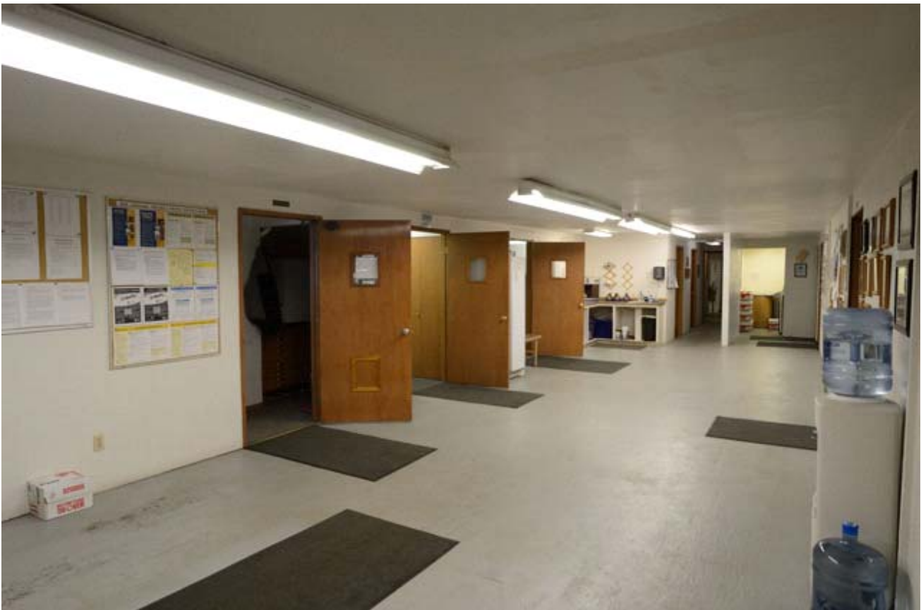
48. Second Floor, Hallway, View Southeast
