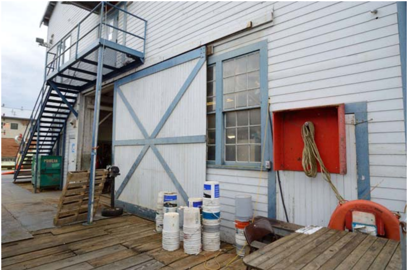
3. Detail of North Elevation, View Southeast
