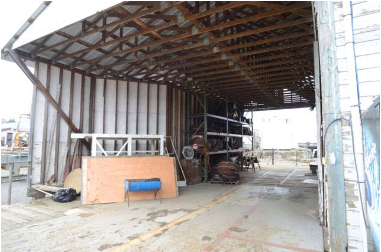
15. Detail of Vestibule Addition, View Southwest
