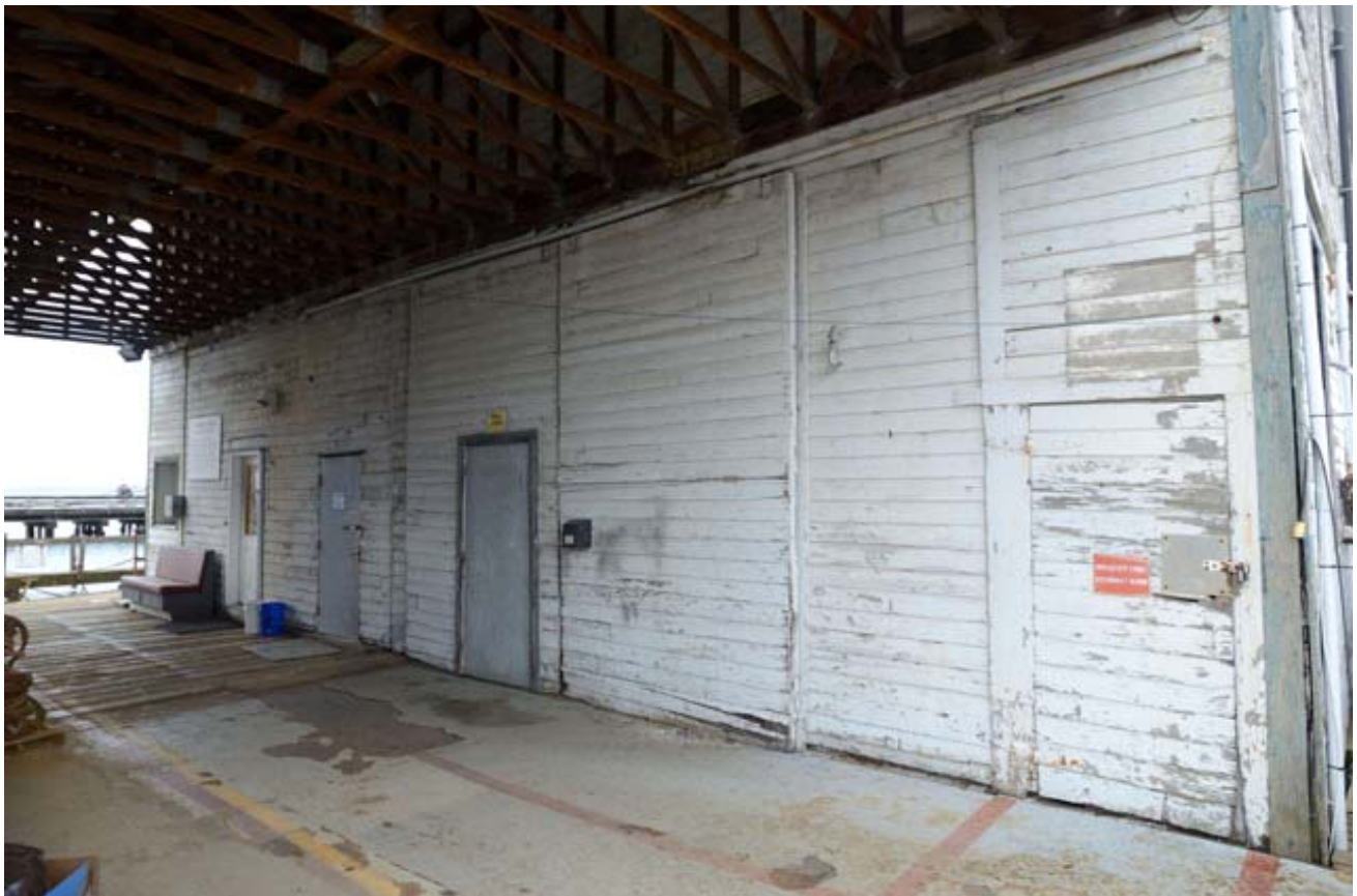
16. Detail of South Elevation, View Northwest
