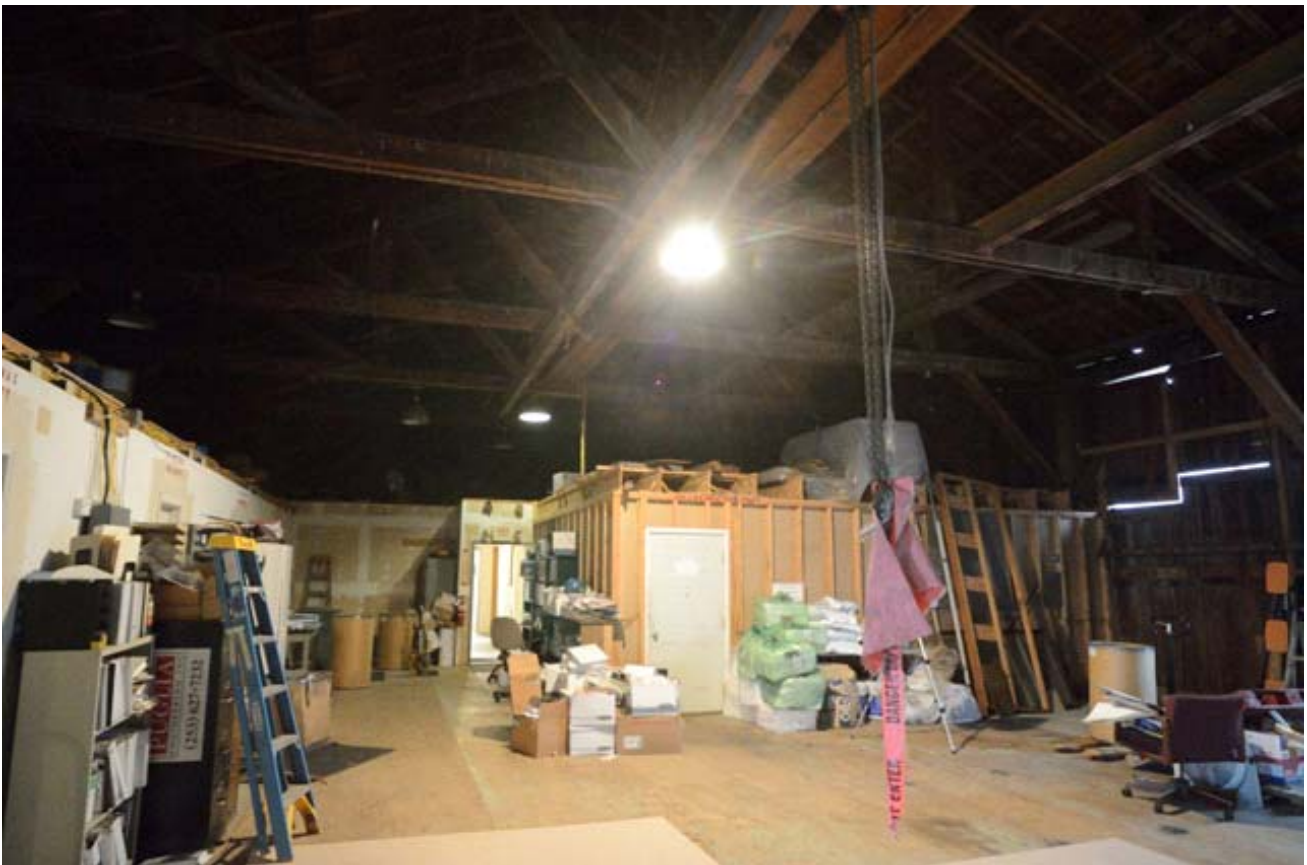
58. Second Floor, Storage Area, View Northeast
