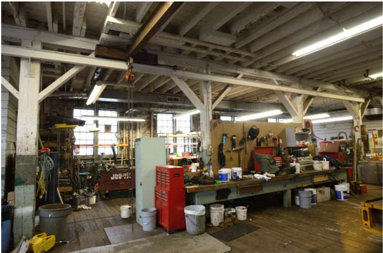
26. First Floor, North Machine Shop, View Southeast
