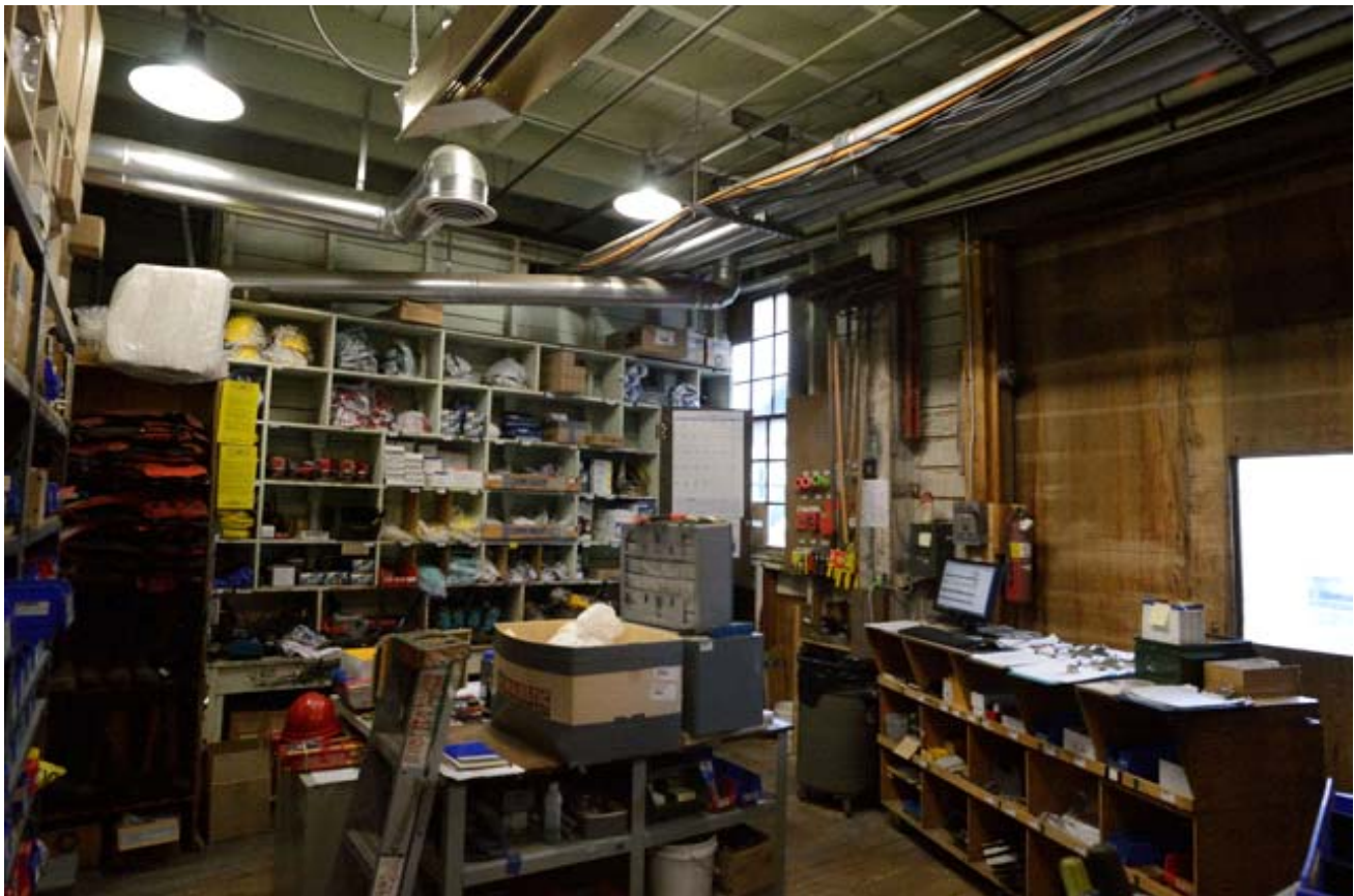
44. First Floor, Supply Room, View Northeast
