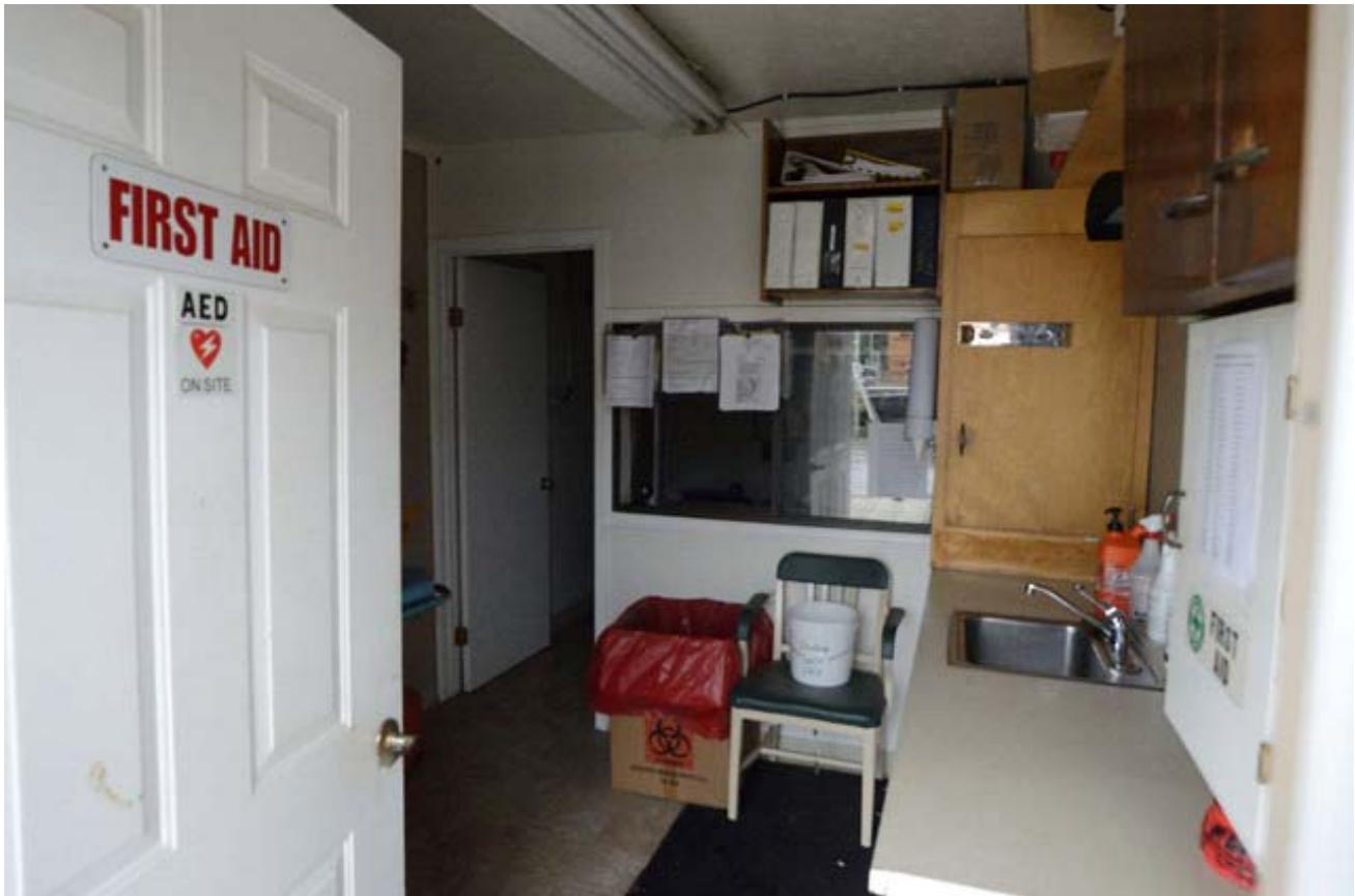
43. First Floor, First Aid Room, View West
