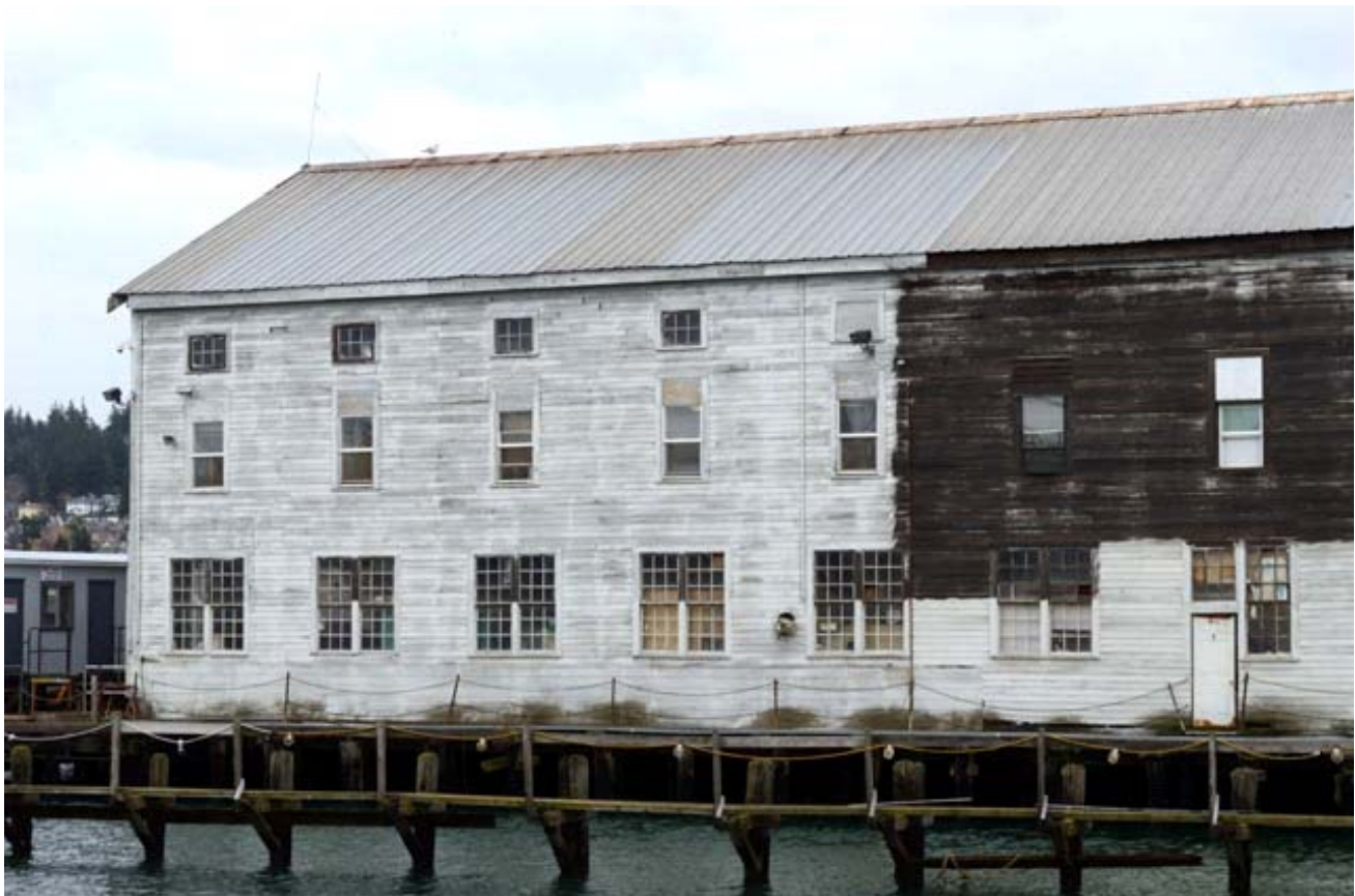
24. Detail of East Elevation, View East
