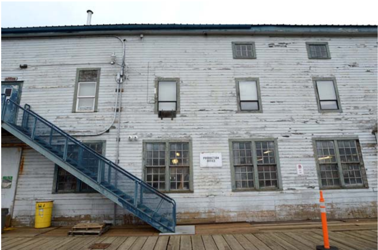
6. Detail of East Elevation, View West
