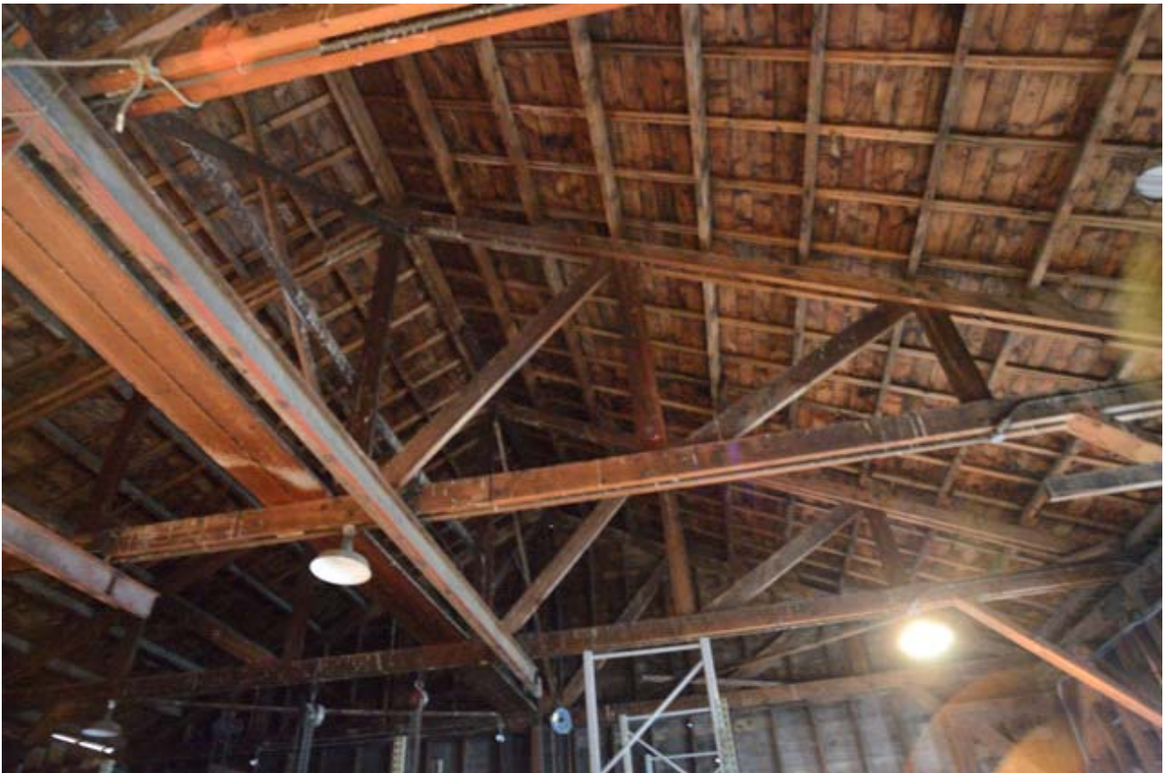
57. Second Floor, Storage Area, View South
