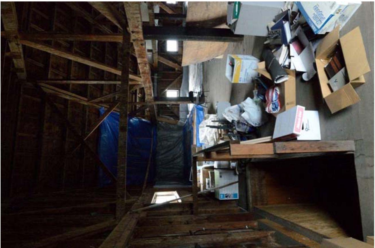
60. Third Floor, View East
