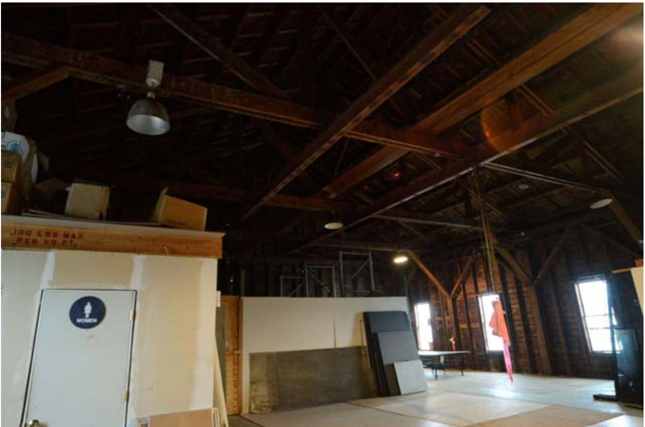
56. Second Floor, Storage Area, View Southwest
