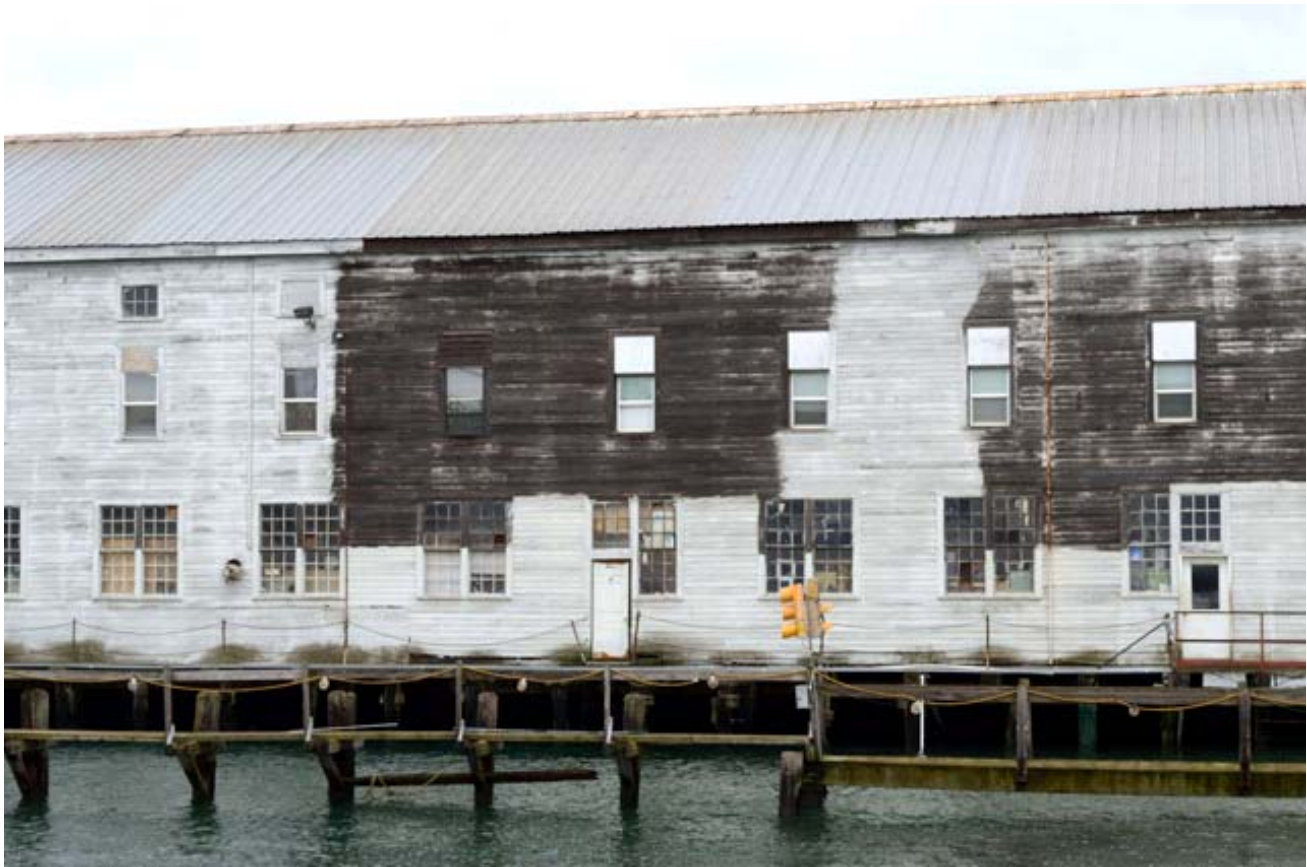
23. Detail of East Elevation, View East
