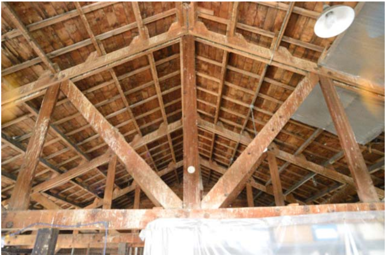
62. Third Floor, View South
