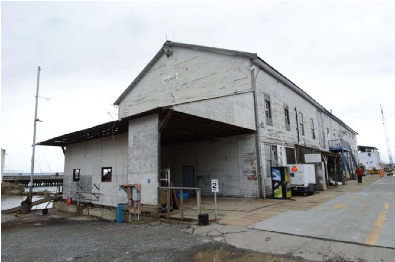
11. South and East Elevations, View Northwest
