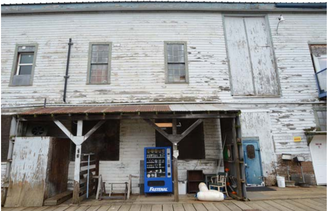
8. Detail of East Elevation, View West
