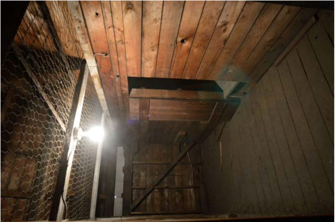
63. Third Floor, View Southeast
