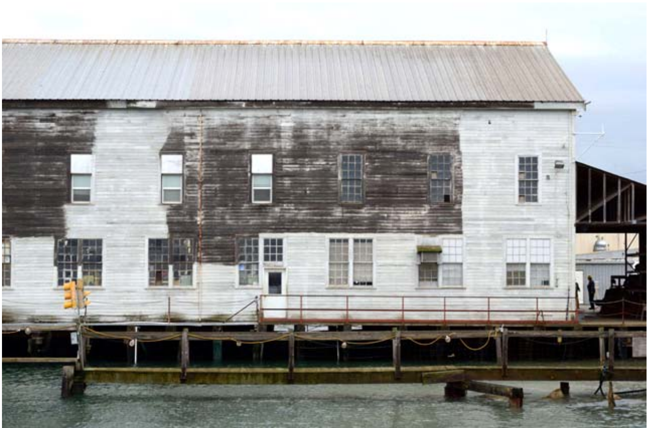
22. Detail of East Elevation, View East
